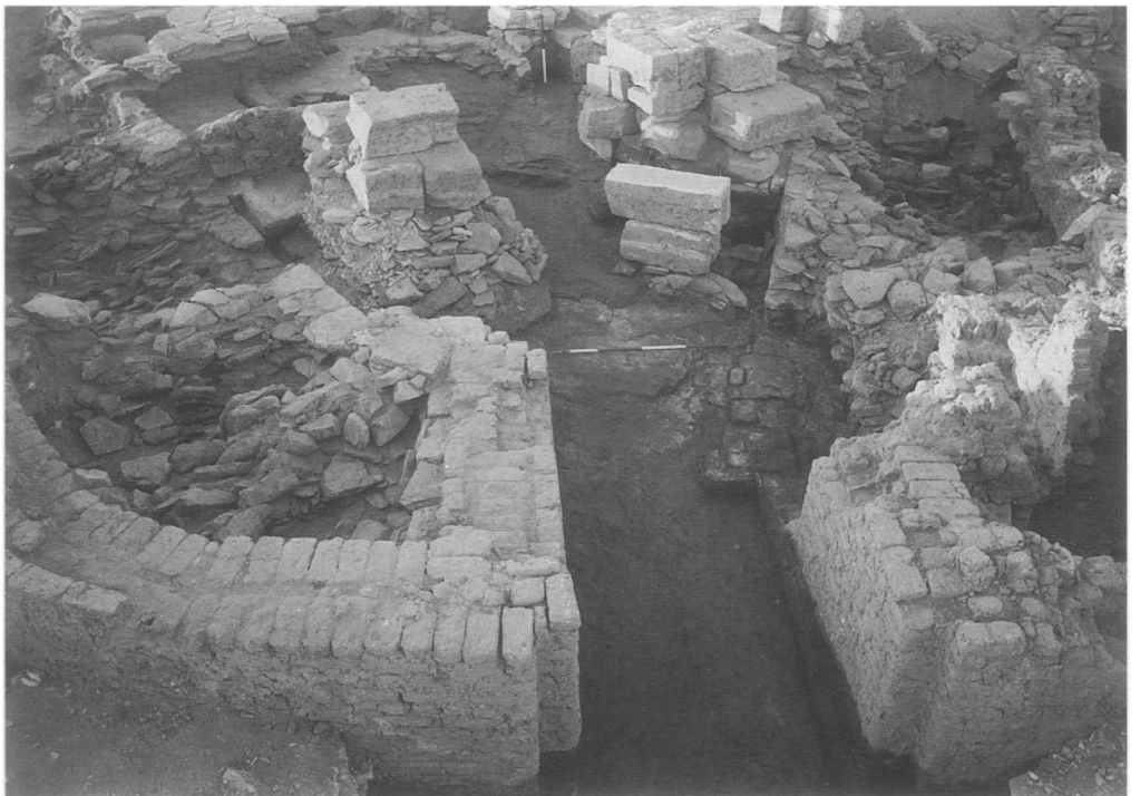
2. The gateway enclosed within the South Bastion looking northwards. The dark area at the bottom of the walls marks the extent of water percolation
